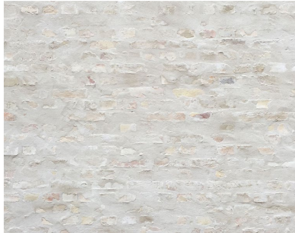
Bagged Brickwork
